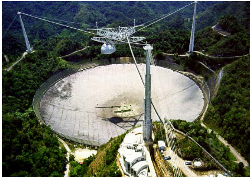
Fig. 3: The Arecibo telescope is a 305 m (1000 feet) diameter spherical reflector, 167 feet deep, and covers an area of about twenty acres. The surface is made of almost 40,000 perforated aluminum panels, each measuring about 3 feet by 6 feet, supported by a network of steel cables strung across the underlying karst sinkhole.
